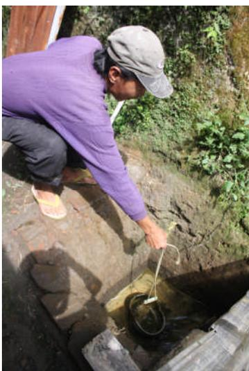
Sludge collection from low-cost community-made biogas plant, powered by animal manure
